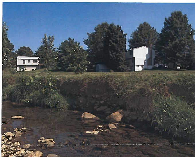
The upcoming NPDES general permit requires MS4 municipalities to develop pollutant reduction plans if they discharge runoff to impaired waters that don't have an established pollution limit.
